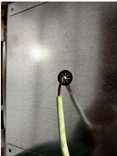
Insert wire through grommet into box:
