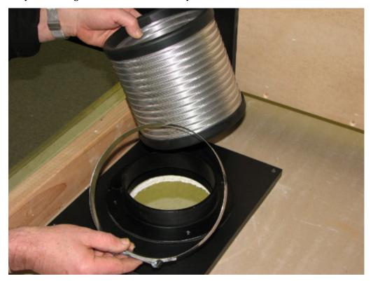
The snorkel expands over a fairly wide range. It should be lengthened until is it slightly taller than is needed for the joists in your installation. If your attic has joists that are smaller than  $2'' \times 8''$ , you may need to trim the aluminum to a more suitable length using a utility knife.
