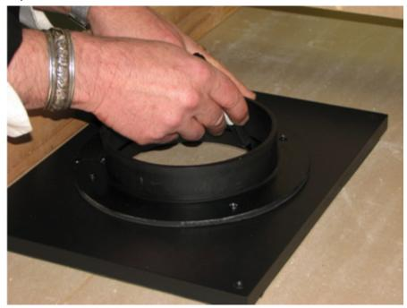
3) Screw the ceiling flange in its location.
